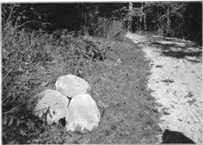
THE DRAINS CONCEALED BY BOULDERS
